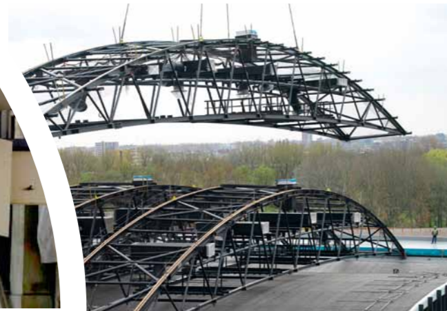
SPORTS HALL AHOY Location: Rotterdam (NL) Tonnage: 1.500 Client: Ahoy - OBR
