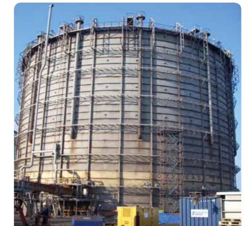
OXY GASHOLDER Location: IJmuiden (NL) Tonnage: 200 Client: Tata Steel
