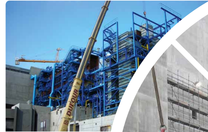
INCINERATOR Location: Dunkirk (FR) Tonnage: 500 Client: Von Roll - Inova
