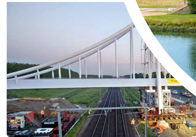
VIADUCT WESTERGO Location: Zoetermeer (NL) Tonnage: 825 Client: Pro Rail
