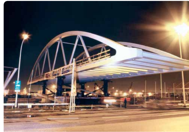
HSL BRIDGE Location: Antwerp (BE) Tonnage: 400 Client: NMBS - Besix
