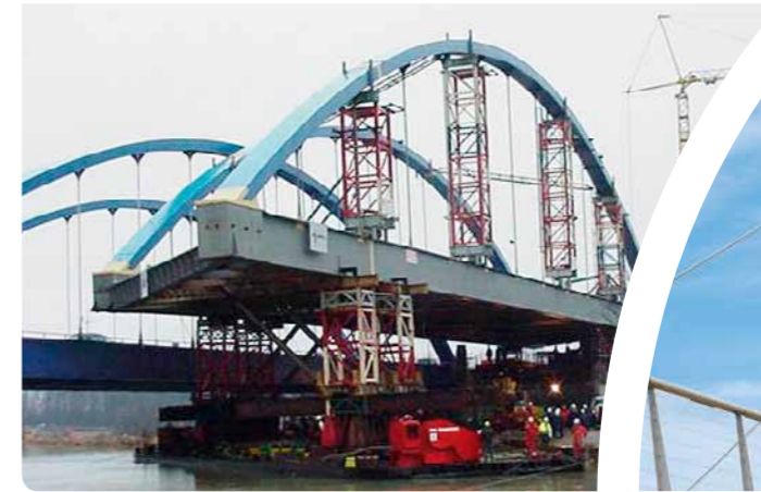
LADBERGEN Location: Ladbergen (DE) Tonnage: 1.050 Client: Ewald Jüchter
