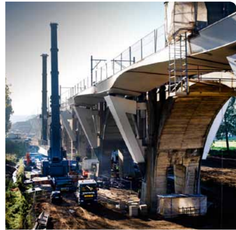
PEDEVIADUCT Location: Dilbeek (BE) Tonnage: 10.000 Client: THV Iemants - Franki - Infrabel
